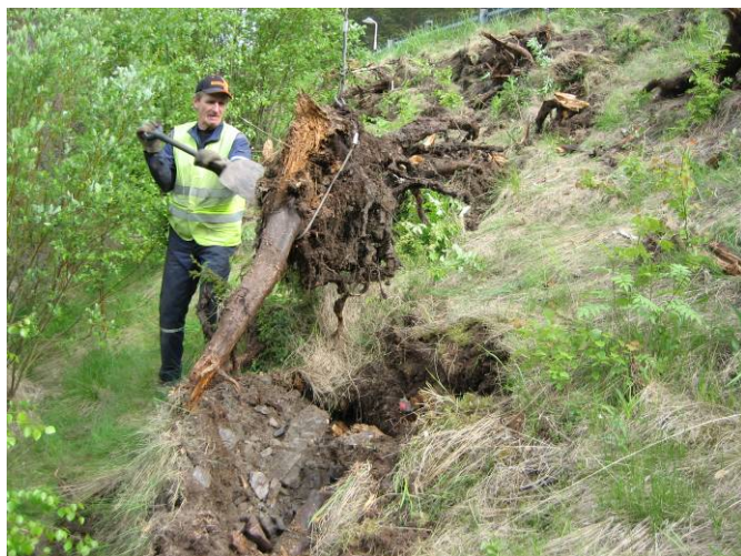
Figure 4: 20-year old pine stump was removed with wire rod at Nuojua.
