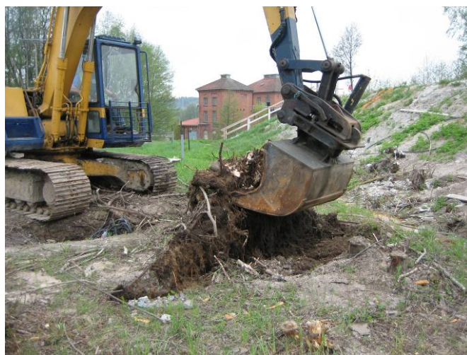
Figure 2: The stump pull test at Peltokoski embankment dam.
