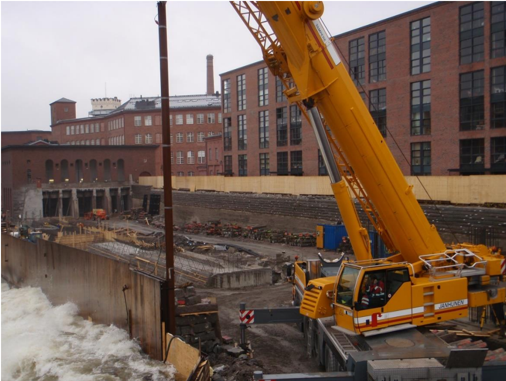
Figure 4: Tammerkoski renovation works – river / canal wall (4.10.2011).
