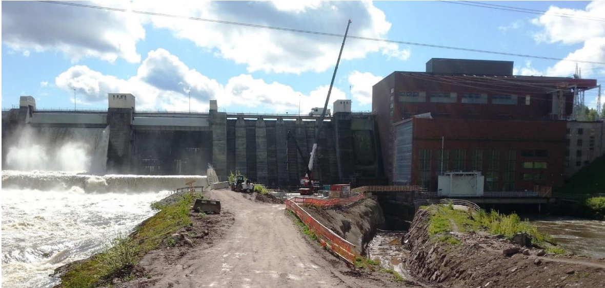
Figure 3. Harjavalta renovation works. (Twitter.com/Harjavaltahydro 28.5.2015)
