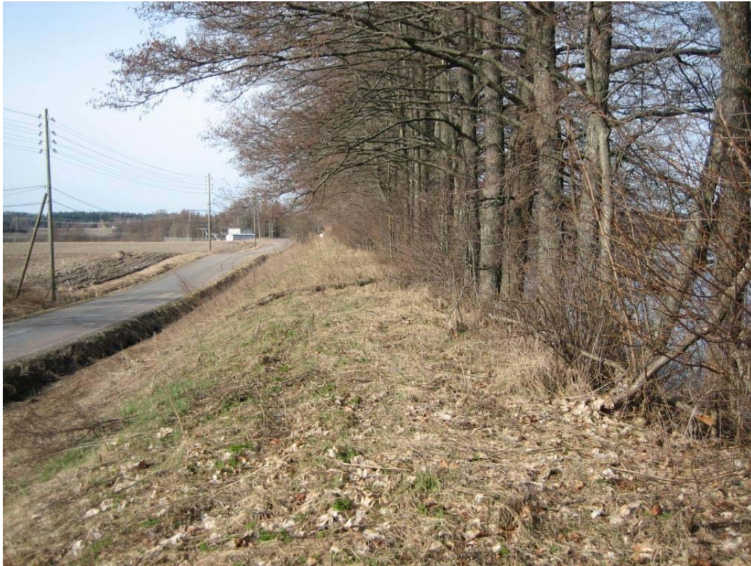
Figure 2. A small embankment with narrow crest width and a trees on the upstream slope.
