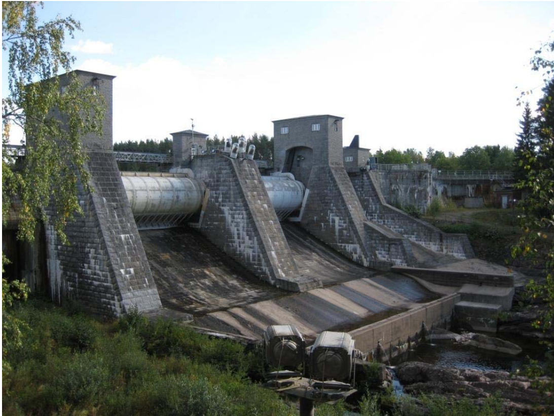
Figure 1. Imatra spillway dam with a roller gates. The construction of the dam was completed in 1929. The hydropower plant has a capacity of 178 MW.
