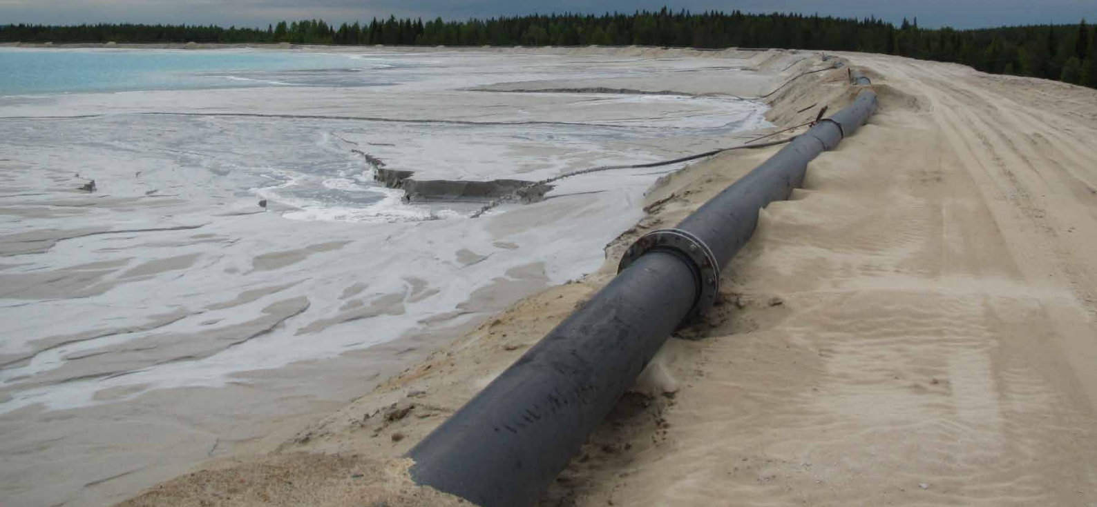
Tailings dam raised using tailings sand, 2012 (Timo Regina)
