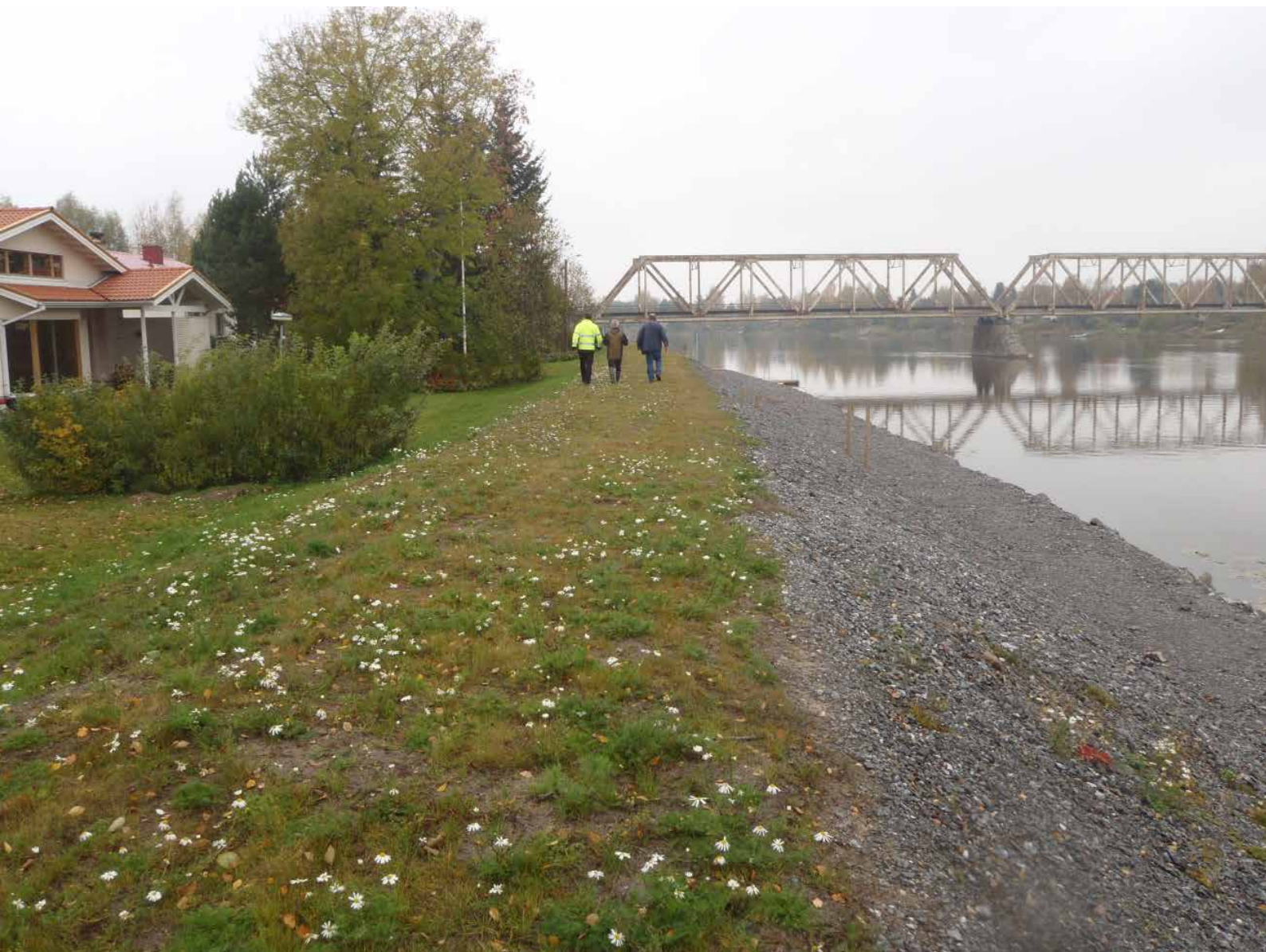
Repaired flood embankment, Pori, 2010 (Milla Torkkel)
